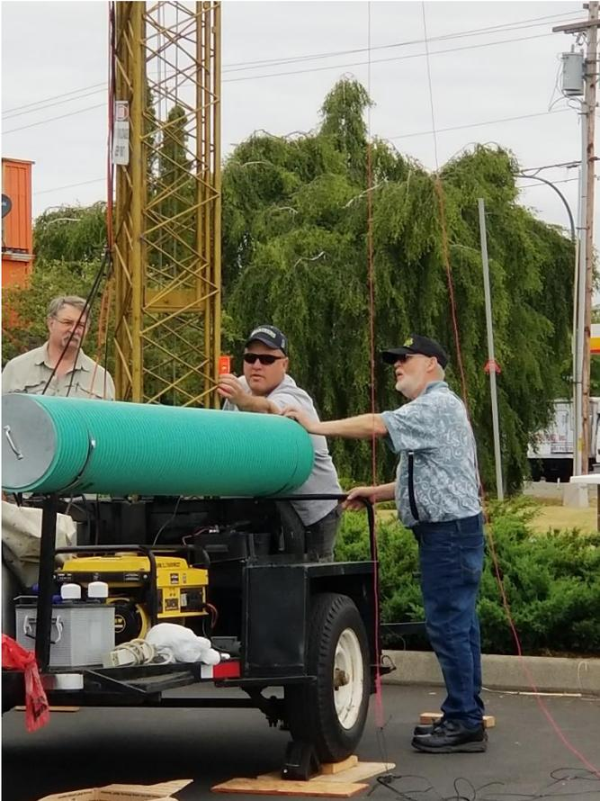
Dale once again allowed us the use of his tower trailer. Several members of the group assisted with the positioning, leveling and raising of the tower. Two inverted V antennas were run on the tower – One 40 meter and one G5RV.
